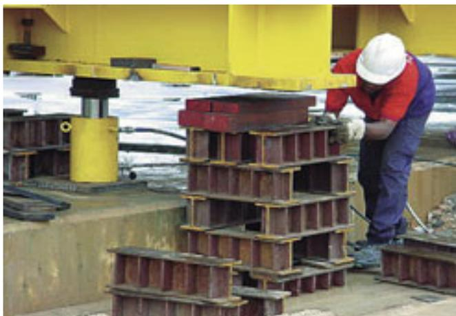
transporting and installing two turbo compressors, each weighing 300 MT with dimensions of 27 M length, 15.50 M height and 7.15 M width, was due to meticulous planning and stringent safety precautions and procedures.
